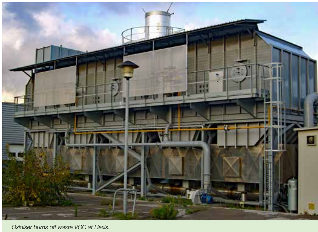
Oxidiser burns off waste VOC at Hexis.
